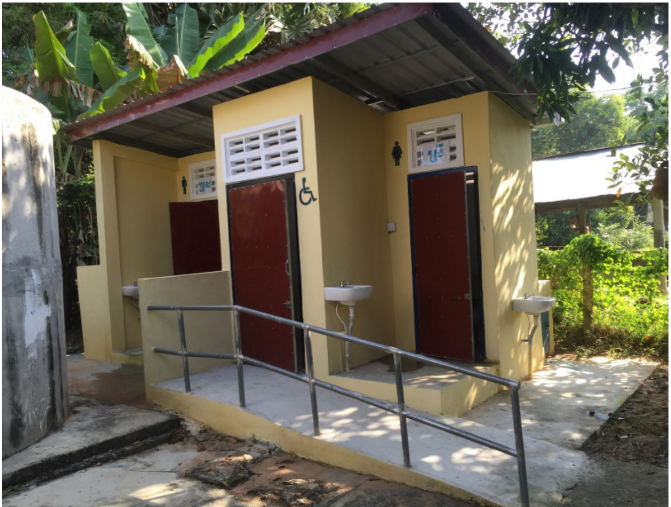
Figure 7: Existing situation of concrete ramp access to toilet
