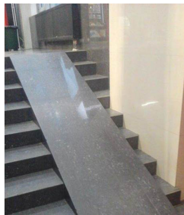
Excessive Steepness of Ramps
