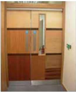
Door-closing devices Some doors in nearly all non-domestic buildings will be required to self-close, including all fire-resisting doors, main entrance and lobby doors, and doors
