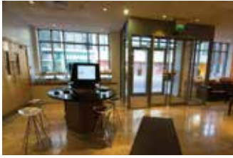
Picture 1.7.1.2. Example of sliding automatic door of entrance lobby
