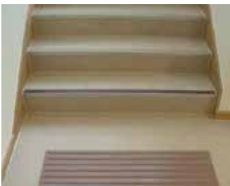
Picture 1.2.5.1. Example of tactile paving surface used as a detectable warning at beginning and the ending of interior stairs
