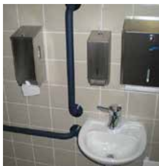
Picture 5.2.1.5. Sample of washbasin with multi-function water tap, soap dispenser, tissues, and handle
