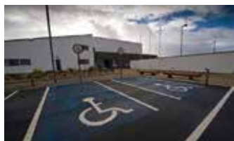
Picture 2.3.6. Sample of design arrangement for appropriate parking space for persons with disabilities
