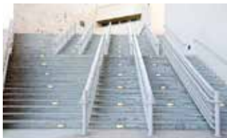
Picture 1.2.4.4. Example of each step of the external stairs with handrails
