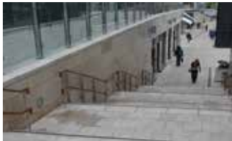
Picture 1.2.4.2. Example of external stairs with stripe surface on top and bottom stair landings and with colored stripes at both handrail and landings
