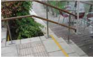
Picture 1.2.4.1. Example of corduroy (tactile) paving at the top of the stairs and double handrails with contrasting color.
