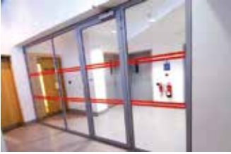
Picture 1.9.1.1. Example of entrance doors
