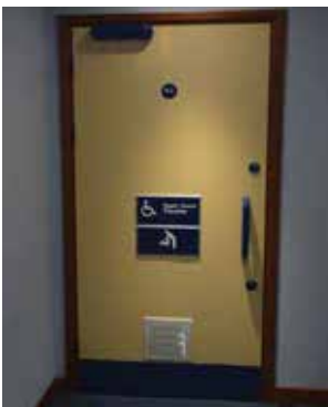
Picture 5.2.1.1. Sample of accessible unisex toilets with sign
