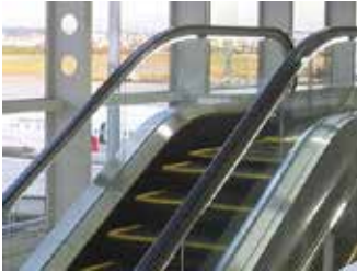
Picture 1.2.9.1. Example of escalator equipped with light on moving handrails
