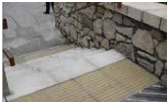
Picture 1.2.4.3. Example of preparation of corduroy (tactile) paving surface for persons with visual impairment, at the beginning and the end of the external stairs
