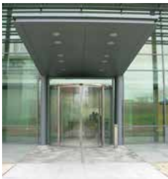
Picture 1.7.1. Example of an entrance to a building
