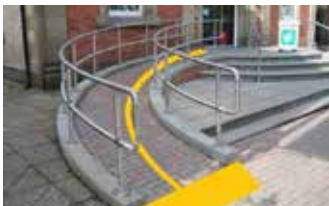
Picture 1.2.1.3. Drawing of ramps with tactile surfaces that can be used by blind people
