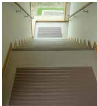
Picture 1.8.1. Example of the corduroy paving areas for people with visual impairment at the beginning and end of the stairs
