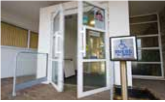
Picture 1.9.5.8.1. Example of two doors opening in and out at the entrance
