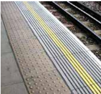
Picture 1.6.1.6. Example of round brown blister and corduroy paving surface
