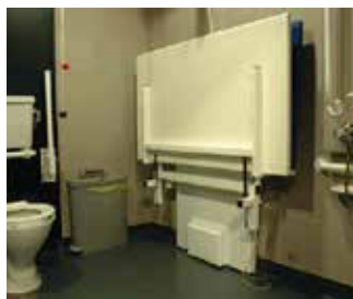
Picture 5.3.2.2. Sample of unisex peninsular-arrangement toilet with assisted changing
