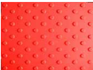
Picture 1.6.1.1. Example of red bricks used for crossing points with traffic light
