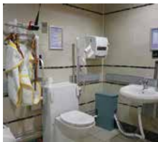
Picture 5.3.2.1. Sample of unisex peninsular-arrangement toilet with hoist facilities for persons with disabilities
