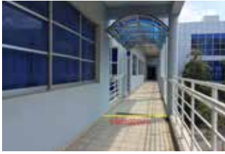
Picture 1.8.1.3. Example of corridor in the upper floor building where two wheelchairs can avoid each other
