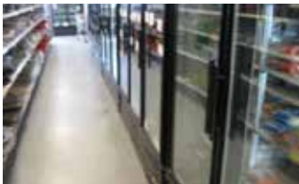
Picture 3.3.2.2. Shows the front view of refrigerators at shopping center
