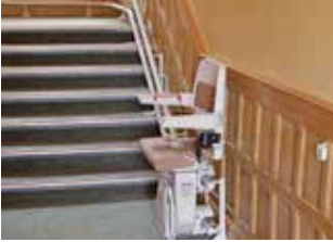
Picture 1.2.8.1. Example of a stair lift: A fixed seat attached to handrail
