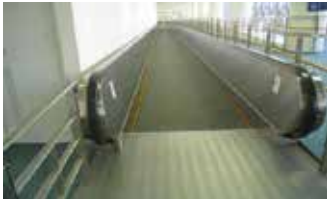
Picture 1.2.10.1. Example of travelator
